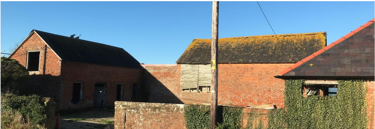
Barns at Glebe Farm (conversion) – WSG007
