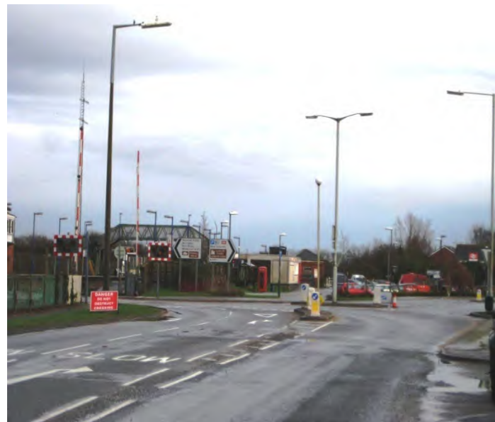
3. The northern entrance to Wool via the A352 and level crossing is a highway dominated space and a poor gateway.
