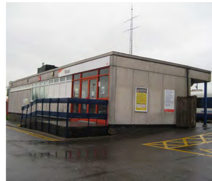
fig. D. The original station was demolished in 1969 and replaced with the current one, seen here.
