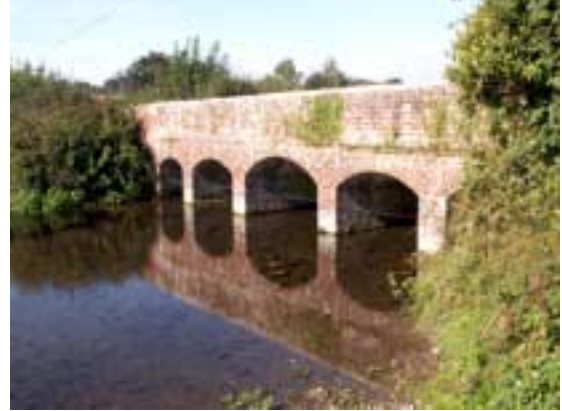
Bridge near French's Farm, Grade II Listed
