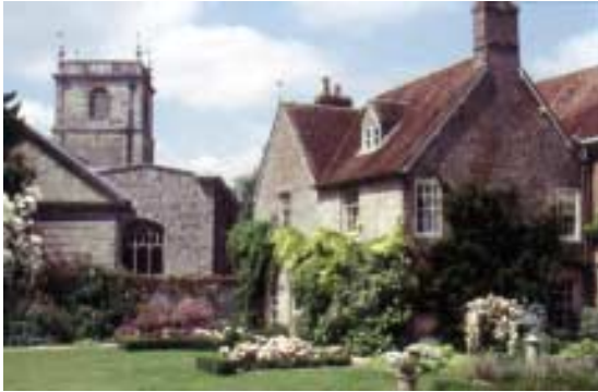
The Rectory, a Grade II Listed Building
