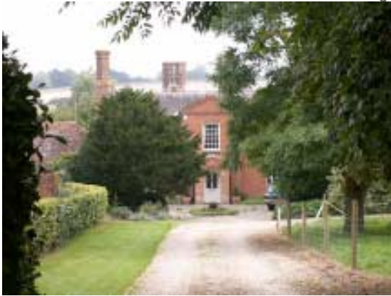
All Hallows Farmhouse, a Grade II Listed Building
