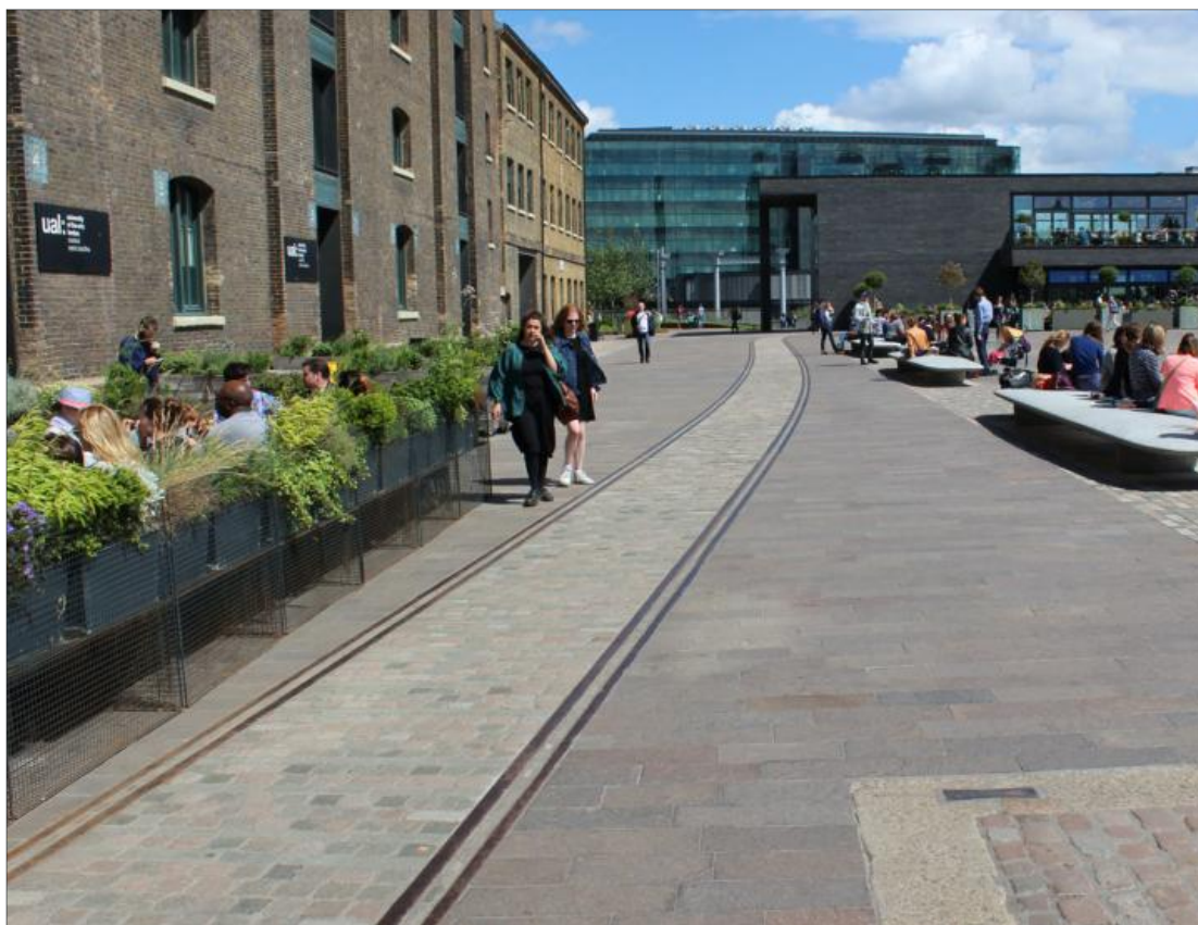
Figure 25 –Example of Infilled Rail Tracks in the Public Realm, King’s Cross, London
