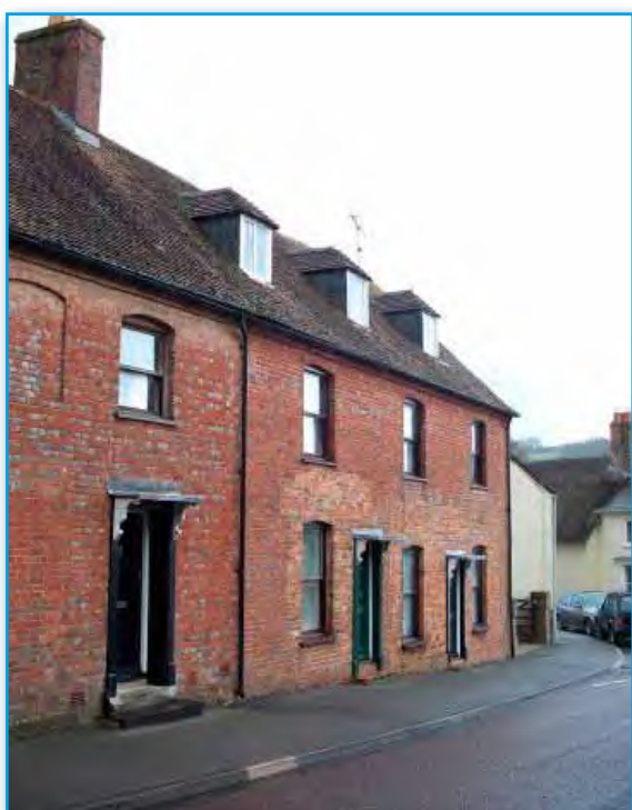
Dormer windows. Careful compositions using hipped roof dormers in Bere Regis and Corfe Castle.
