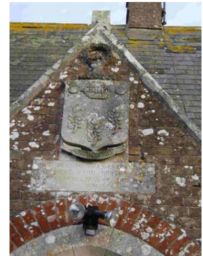
Fig 40. Entrance detail of Primary School
