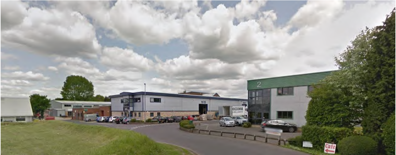
Figure 19. Bailie Gate Industrial Estate
