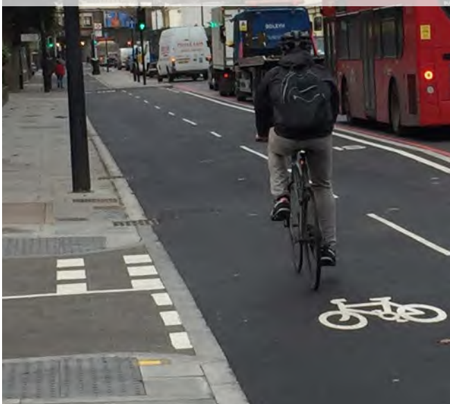
Figure 7.10: Tight kerb radii at residential side street
