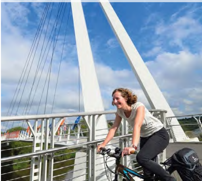
Figure 10.49: Diglis Bridge, Worcester
