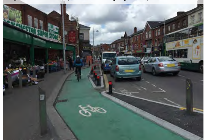
Figure 1.10: Example of kerb-segregated cycle track
