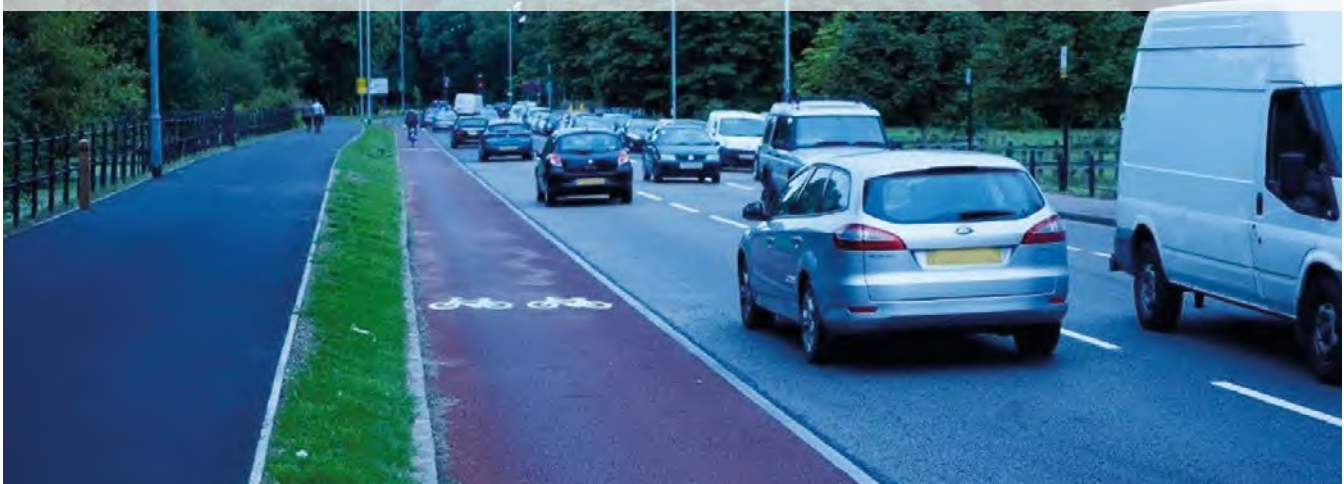
Figure 6.13: Double TSRGD diagram 1057 symbols on one way stepped cycle track, Cambridge
