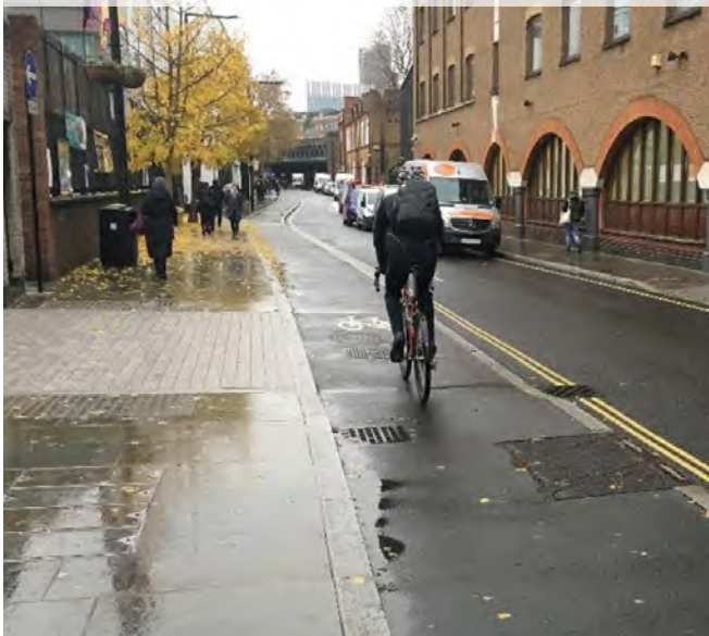
Figure 6.11: Contraflow stepped cycle track, London, showing cycle track draining towards footway
