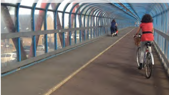
Figure 10.50: Covered pedestrian/cycle bridge across railway tracks, Cambridge
