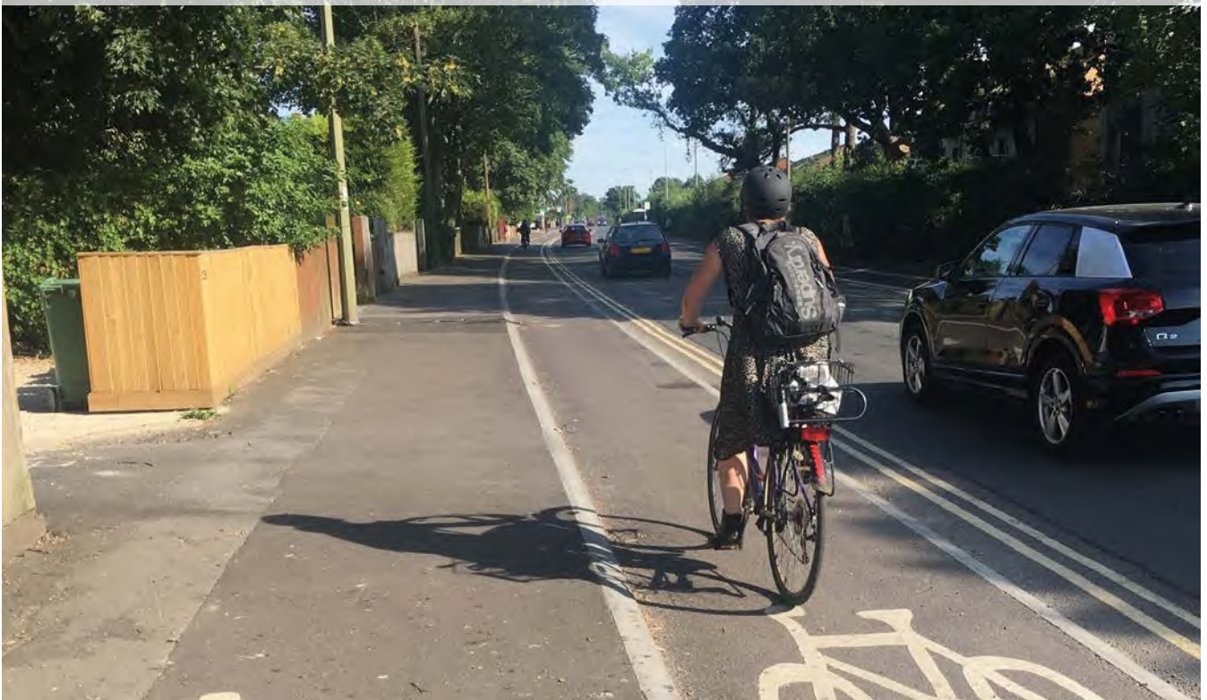
Figure 4.3: Edge of city distributor road, Oxford uses a stepped cycle track for separation from motor traffic
