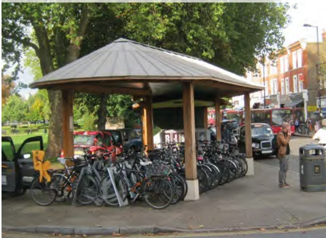
Figure 11.10: Small cycle hub at Ealing Broadway offering CCTV secure parking and cycle hire
