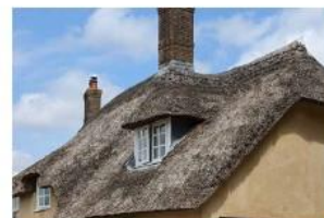
Half hipped thatched roof with hipped dormers
