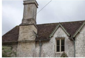
Chimney and gabled dormer
