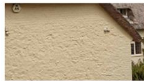
Painted brick and part plastered cob
