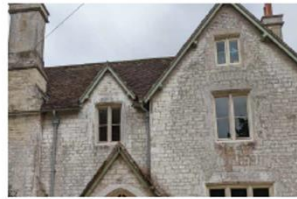
Red clay tiles on a gabled (& cross gabled) roof
