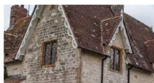
Rough ashlar wall with stone mullioned window
