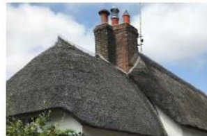
Thatched gabled roof with brick chimney
