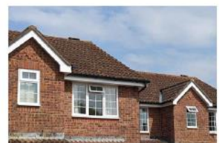
Clay tiles on cross gabled roof
