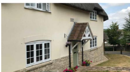
Figure D: Pitched roof canopy porch, West Stafford.
