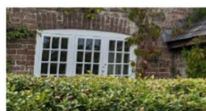
Casement windows (painted white)
