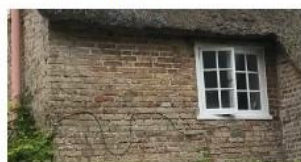
Brick walls in English bond
