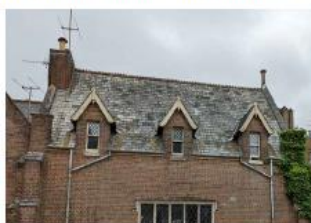
Pitched roof with dormers.
