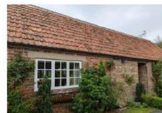
Light red/ orange, clay pantiles on a gabled roof
