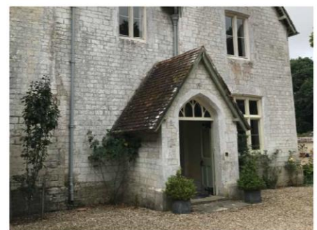
Figure F: Enclosed, pitched roof front porch, Woodsford.
