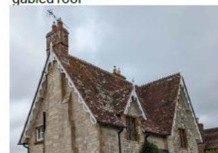
Gabled (and cross gabled) roof with decorative roof detailing and dormers
