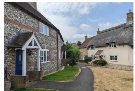
Figure C: Open pitched roof porch (foreground) and pentice canopy porch (background), West Stafford.
