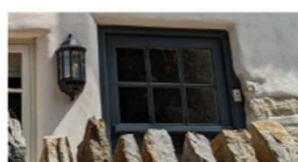
Casement windows (painted blue)
