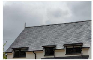
Grey slates on gabled roof
