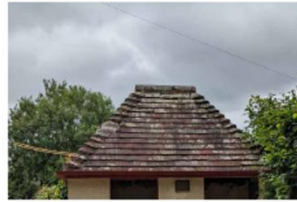
Clay tiles on bonnet tiled hipped roof
