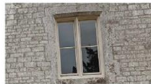
Painted timber frame on sash
