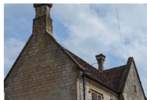
Clay tiles on cross gabled roof with brick chimneys
