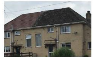
Hipped roof with clay tiles
