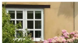
Modern casement windows
