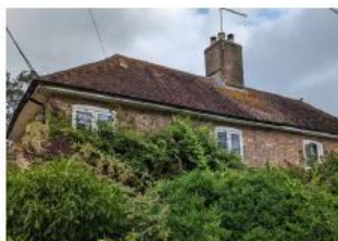
Red, clay pantiles on a hipped roof
