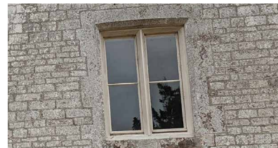
Painted timber frame on sash windows
