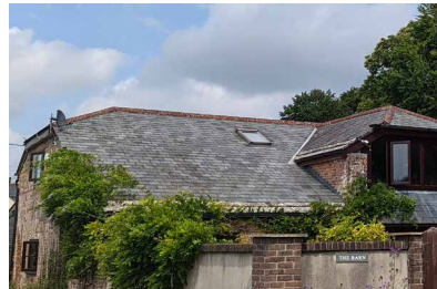
Grey slates on half-hipped roof with hipped dormer
