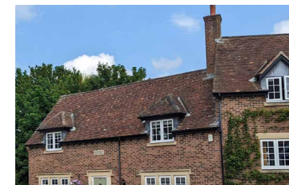
Gabled roof with clay tiles and hipped dormers
