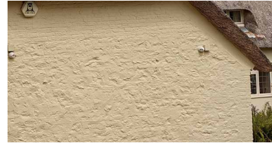
Painted brick and part plastered cob
