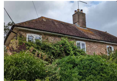
Red, clay pantiles on a hipped roof
