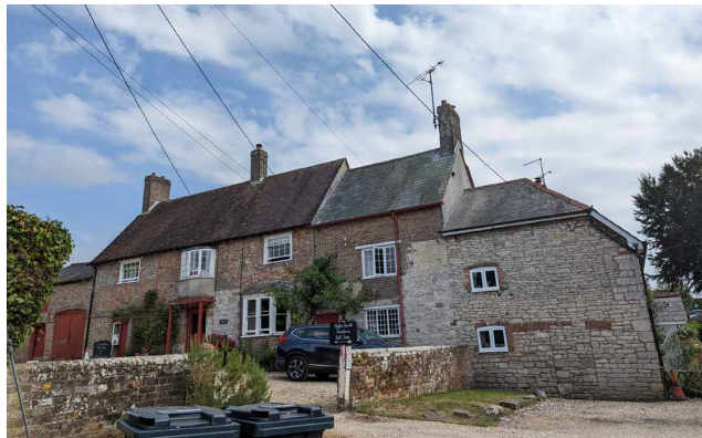
Figure 26: Grade I listed Woodsford Castle (top photo) and Grade II listed Higher Lewell farmhouse (bottom photo). Any new development in close proximity to listed buildings should sit sensitively next to them respecting their scale and massing while allowing for a generous setback.
