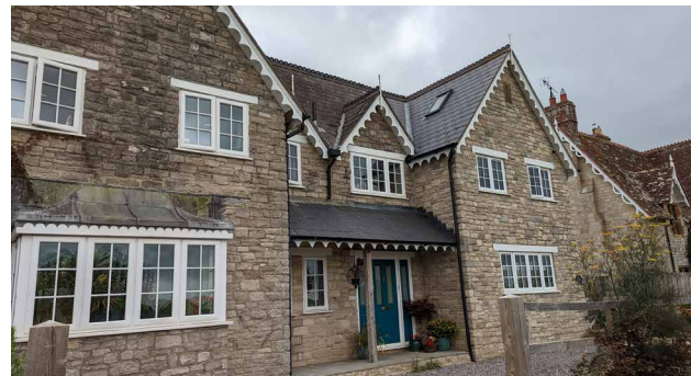
Figure 40: Decorative ridge tiles, decorative eaves and pentice porch, Tincleton.
