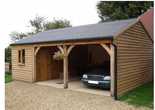
Figure 70: Example of a car barn as a recommended alternative for parking solution.
