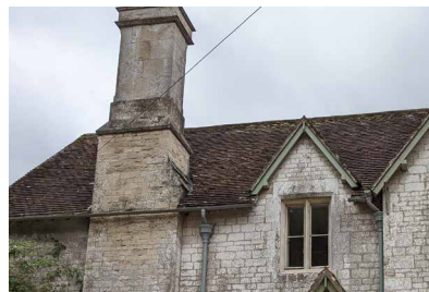
Chimney and gabled dormer
