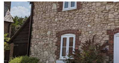
Limestone and dark red brick around windows and doors
