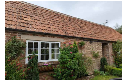
Light red/ orange, clay pantiles on a gabled roof
