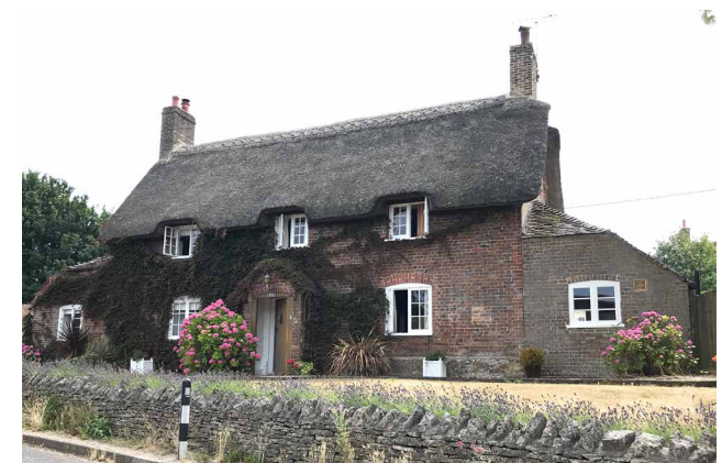
Figure 61: Positive example of a side extension that respects the existing building in terms of scale and building materials, West Stafford.
