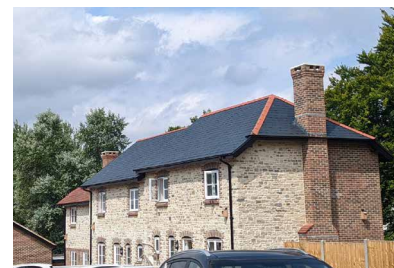
Grey slate tiles on hipped roof with brick chimney on the side
