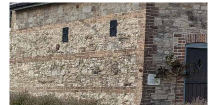
Limestone and dark red brick around windows and doors
