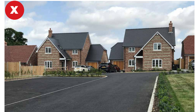
Figure 32: Local example of infill development where architectural details, heights and massing do not entirely match with the surroundings, while the large tarmacked area clashes with the permeable, and earthy palette, surfaces that characterise the rest of the properties in the village, West Stafford.
