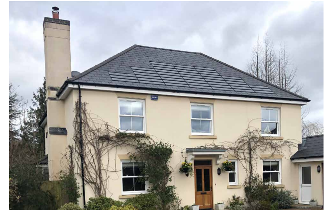
Figure 95: Use of shingle-like solar panels on a slate roof with the design and colour of the panels matching those of the adjacent slate tiles
