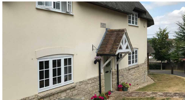
Figure 39: Pitched roof canopy porch, West Stafford.
