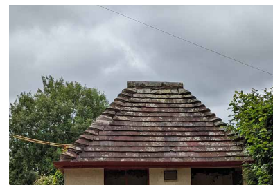
Clay tiles on hipped roof
