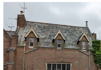
Pitched roof with dormers.
