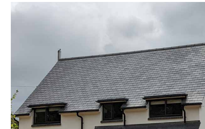
Grey slate tiles on gabled roof
