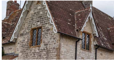
Rough ashlar wall with stone mullioned window
