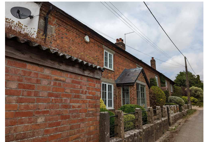
Figure 118: House with a small set back from the road and a combination of brick wall, concrete column and iron railing boundary treatment with additional planting in the front garden.
