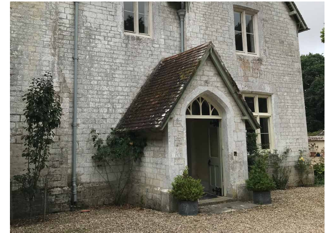
Figure 42: Enclosed, pitched roof front porch, Woodsford.
