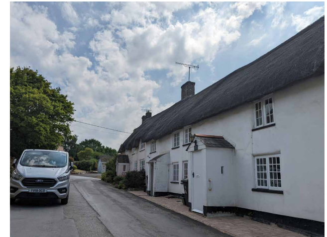
Figure 50: Thatch roofed terraced housing in West Knighton.
