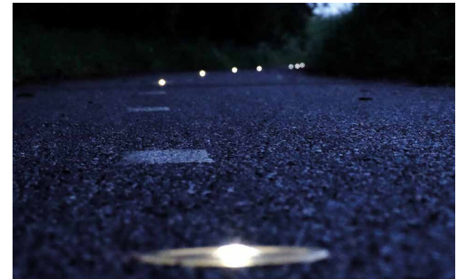
Figure 82: Example of a foot/cycle path which is lit by solar cat's-eye providing some light for pedestrian and cyclists without creating any disturbance to the nearby properties or unacceptable levels of light pollution.
