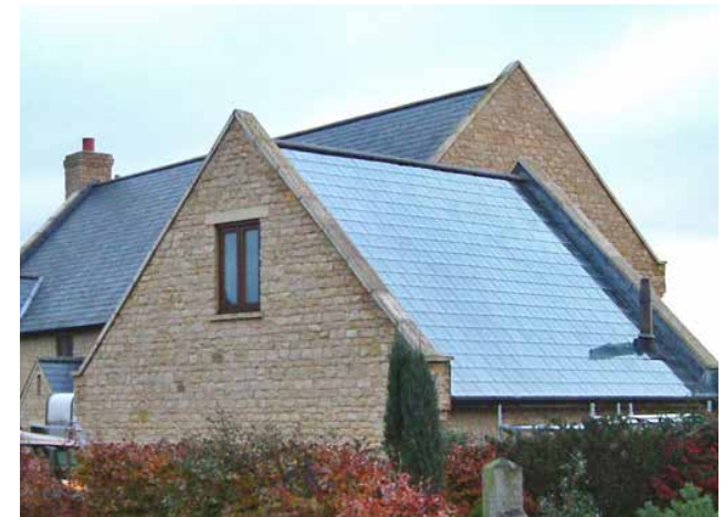
Figure 96: Positive example of implementing solar panels from the design stage.
