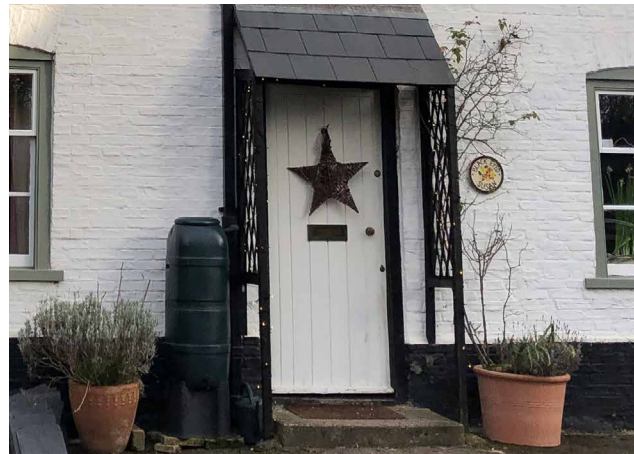
Figure 85: Examples of water butts used for rainwater harvesting in Reach, Cambridgeshire.
