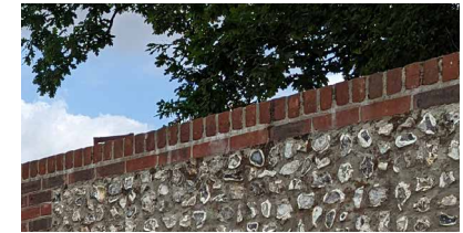
Flint wall with red brick along the edges
