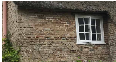
Brick walls in English bond
