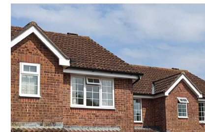
Clay tiles on cross gabled roof
