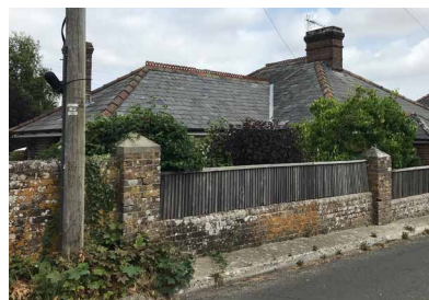
Grey, slate tiles on a hipped (and cross gabled) roof
