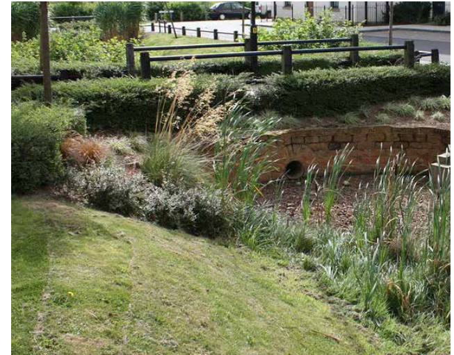
Figure 83: Example of swales check dam integrated with a crossing point, somewhere in UK.
