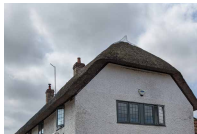
Mansard thatched roof
