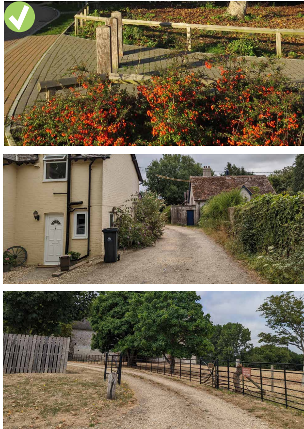
Figure 11: Positive examples of permeable paving. The top photo show examples of paving that could be used within the built environment, while the middle and bottom photos show an example of edge lane that uses gravel, in earthy palette, which could also be used in footpaths within the countryside.
