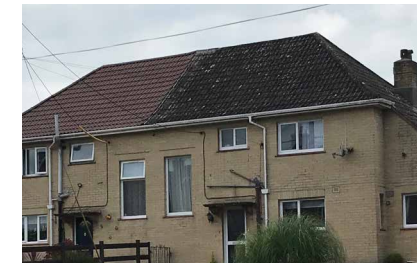
Hipped roof with clay tiles
