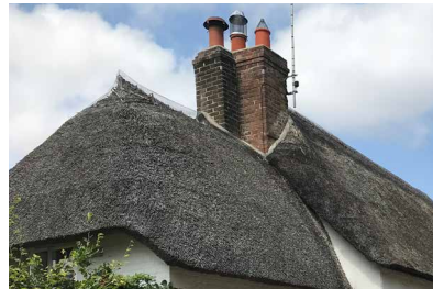
Thatched gabled roof with brick chimney
