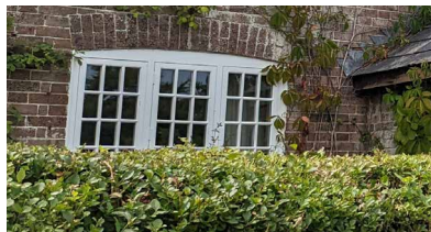
Casement windows (painted white)
