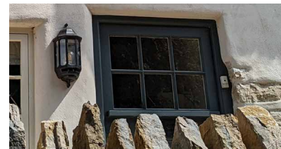
Casement windows (painted blue)
