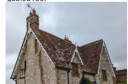
Gabled (and cross gabled) roof with decorative roof detailing and dormers
