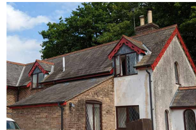
Grey slate tiles on gabled roof with gabled dormer
