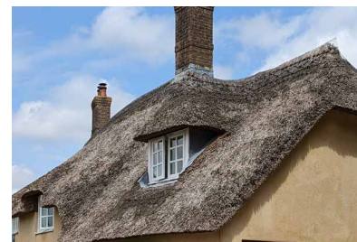
Mansard thatched roof with hipped dormers
