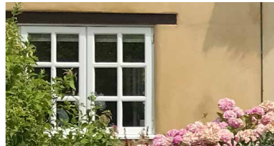
Modern casement windows
