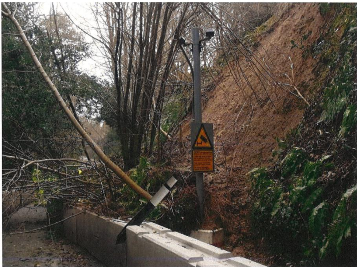
Figure 2: Landslip – viewing North
