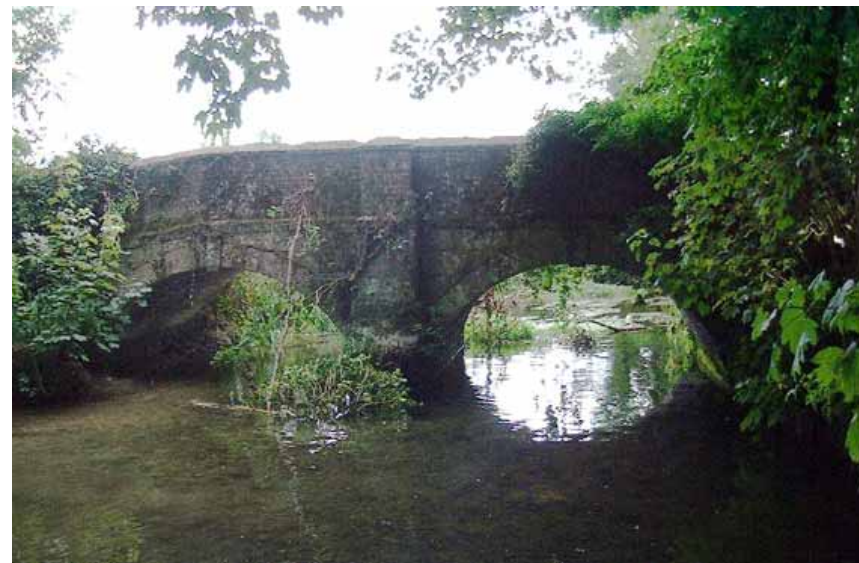
Roadbridge at Witchampton
