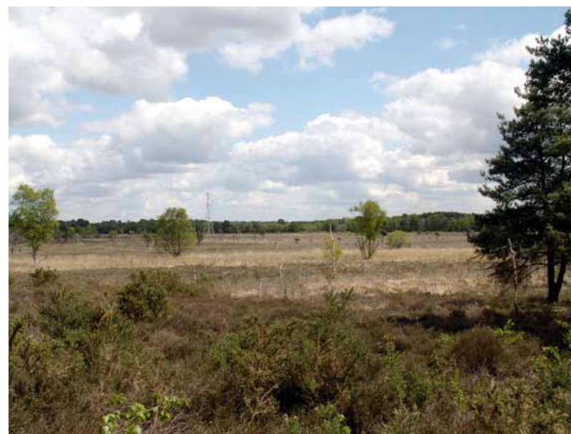
View across southern part of Parley Common with the prominent overhead lines in the background
