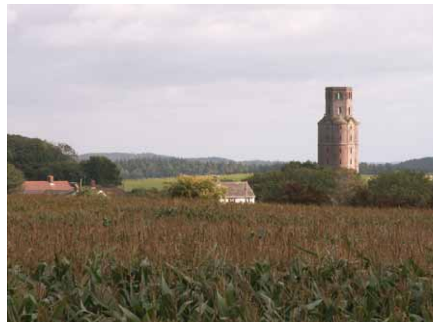
Horton Tower, a Grade II* listed building and a prominent landmark
