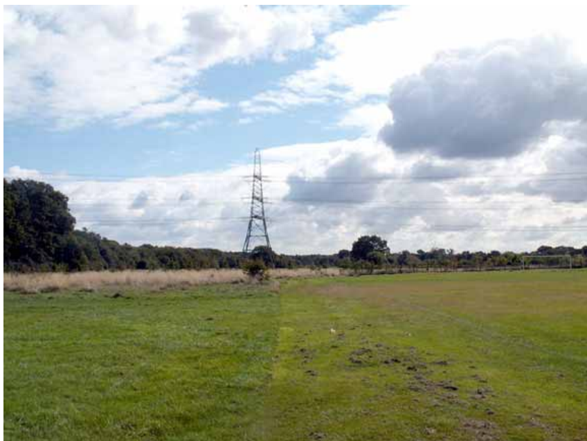
The river terrace at Potterne, Potterne Wood and the river to the left, note the impact of the o/h line in this landscape
