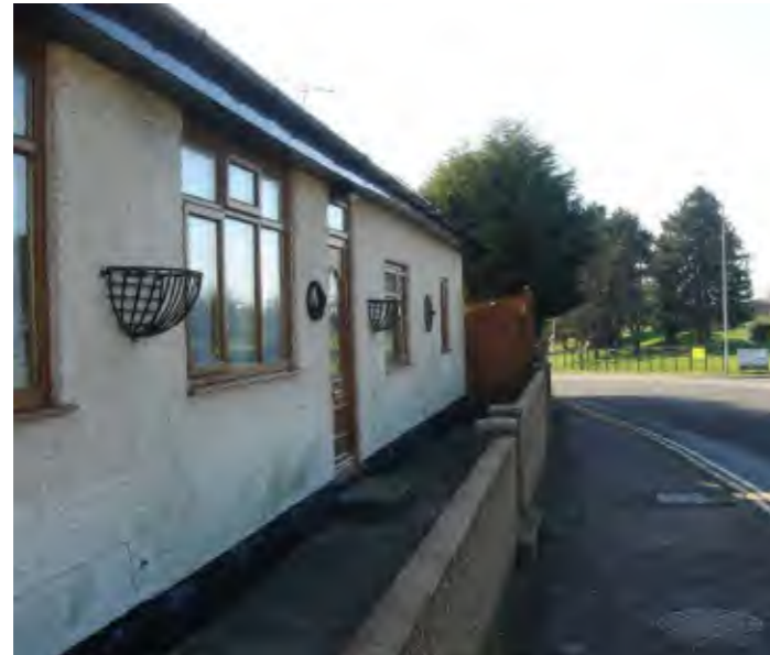
1. Bungalow on King George V Road opposite Bovington First School
