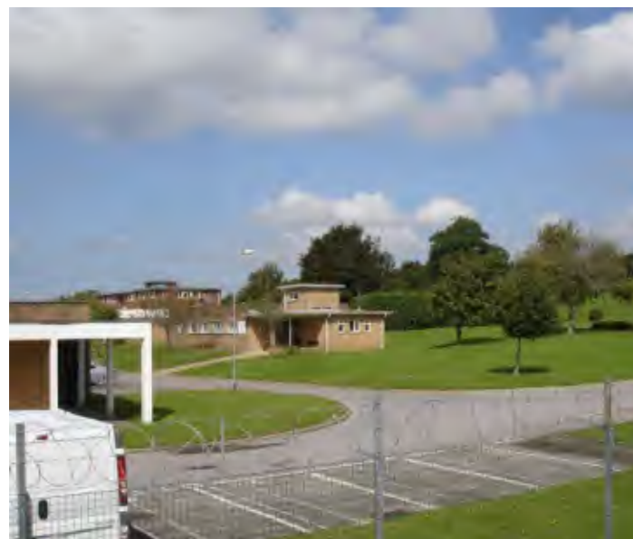
3. An example of the orthogonal layout of the military base at Stanley Barracks.
