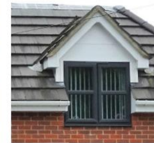
Gable dormer with painted timber casement window.
