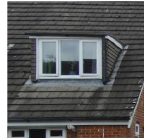
Flat roof dormer with casement windows.
