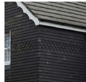
Continuous pattern in weatherboards and decorative fascias.
