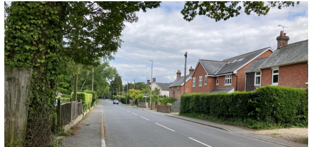
Figure 1. B3078 Station Road, looking east
