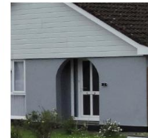
Arched inset front doorway.
