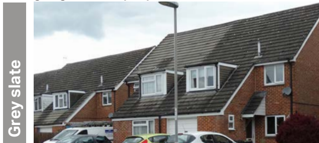
Continuous catslide roof with parallel flat roof dormers.
