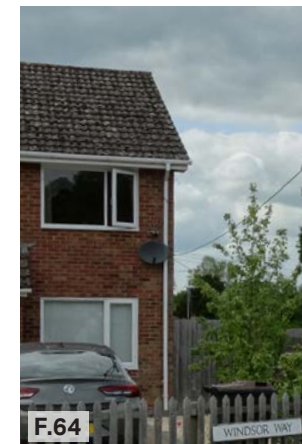
Figure 64: Example of external additions (satellite) that are displayed on the front-facing facade and not placed discretely.
