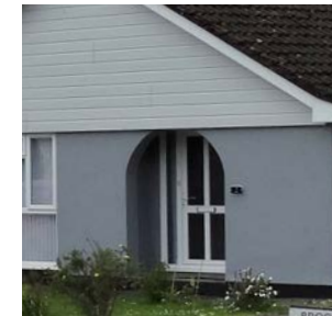
Arched inset front doorway.
