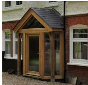
Gable portico with timber frame and glazing.
