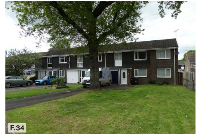
Figure 34: Terraced Housing Along Earlswood Drive.
