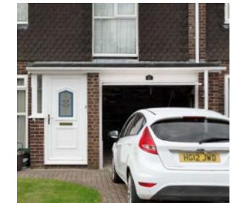
Entryway flat overhang above front door and garage.
