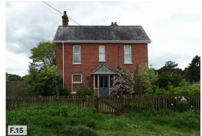
Figure 15: Example of a dwelling located within Character Area 1: Early village footprint.
