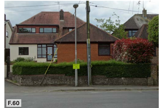
Figure 60: Example of a distinct roof type typically found throughout Alderholt.
