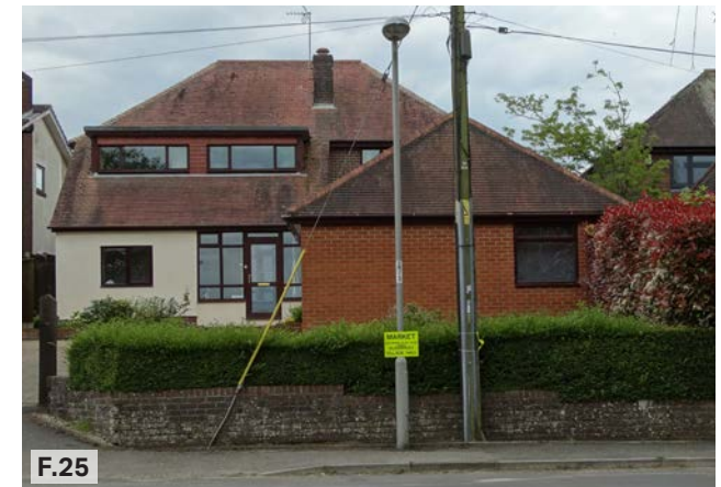
Figure 25: Dwelling along Ringwood Road located on the western edge of the site, featuring a half-hipped roof with red clay tiles and a flat-roof dormer, a light render facade with timber detailing, and a mixed brick and hedgerow boundary treatment.
