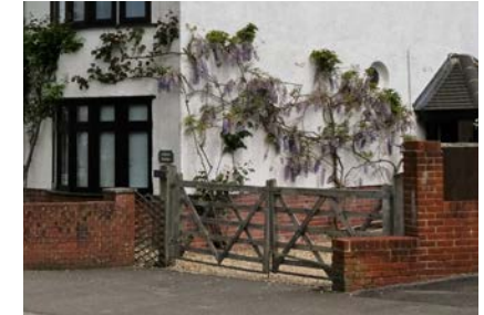
Low brick wall with timber entrance gate.
