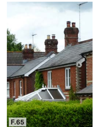
Figure 65: Example of a consistent chimney rhythm with neighbouring dwellings in terms of placement material and scale.
