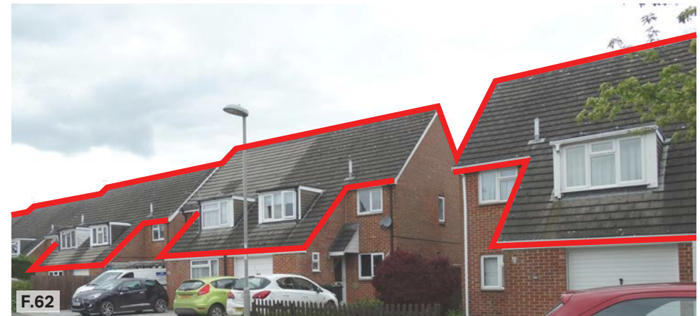
Figure 62: Roofline with consistent style, pattern and features such as scale and placement of dormer windows. This consistency supports a uniform vernacular within specific village areas.
