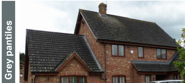
Gable roofs of varying heights with gable dormer and chimney additions.
