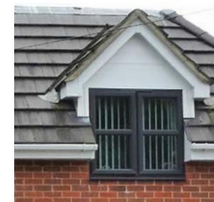
Gable dormer with painted timber casement window.
