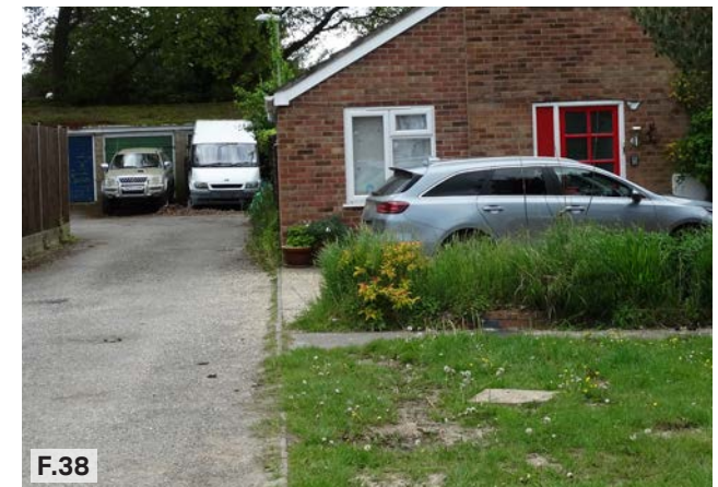
Figure 38: Garage block located behind the building line on Windsor Way.
