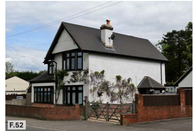
Figure 52: Example of a property with boundary treatments that are fitting with the rural character of Alderholt.
