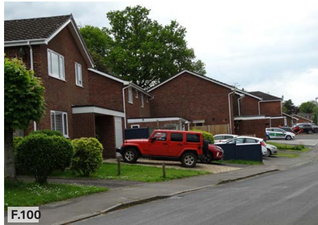
Figure 100: Example of on-plot parking in front of the dwelling.
