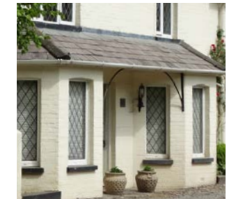
Symmetric bay windows with diamond glazing bar pattern.
