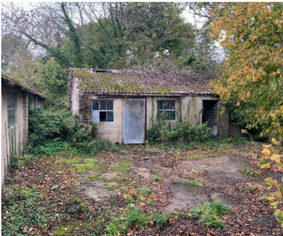
Photo 11 - View from within existing farm buildings yard
