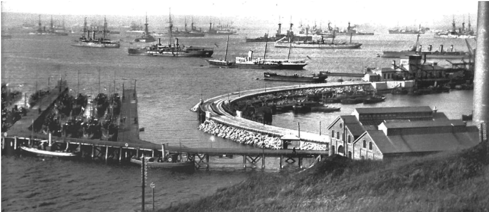
Fig. 14: Portland harbour Review of the fleet, 1912 torpedo boat pens (left) and electricity sub-station and chimney (right). Note transitional form of Royal Navy ships with both masts and steam funnels. (Morris)
