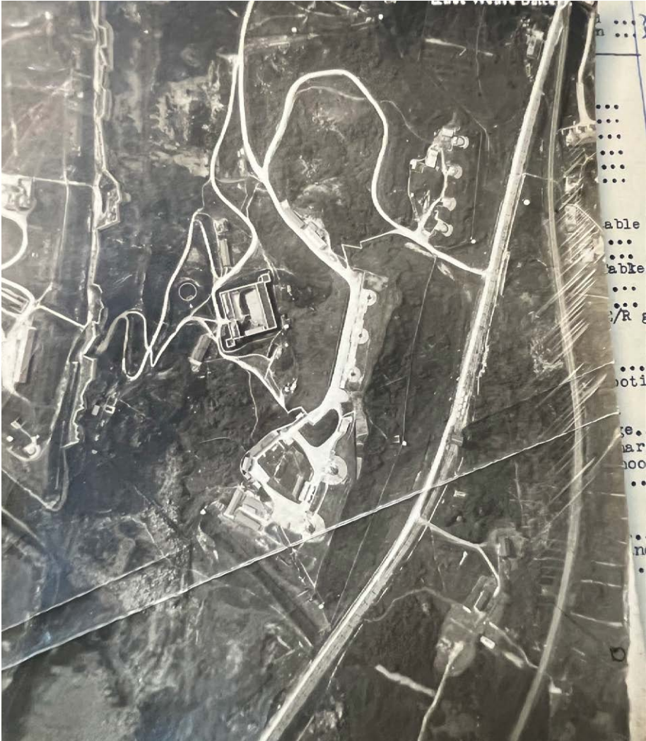
Fig. 16: Fig. 16 Very early 1917 aerial photograph of the Provost Establishment and A and B batteries by the Central Flying School. National Archives
