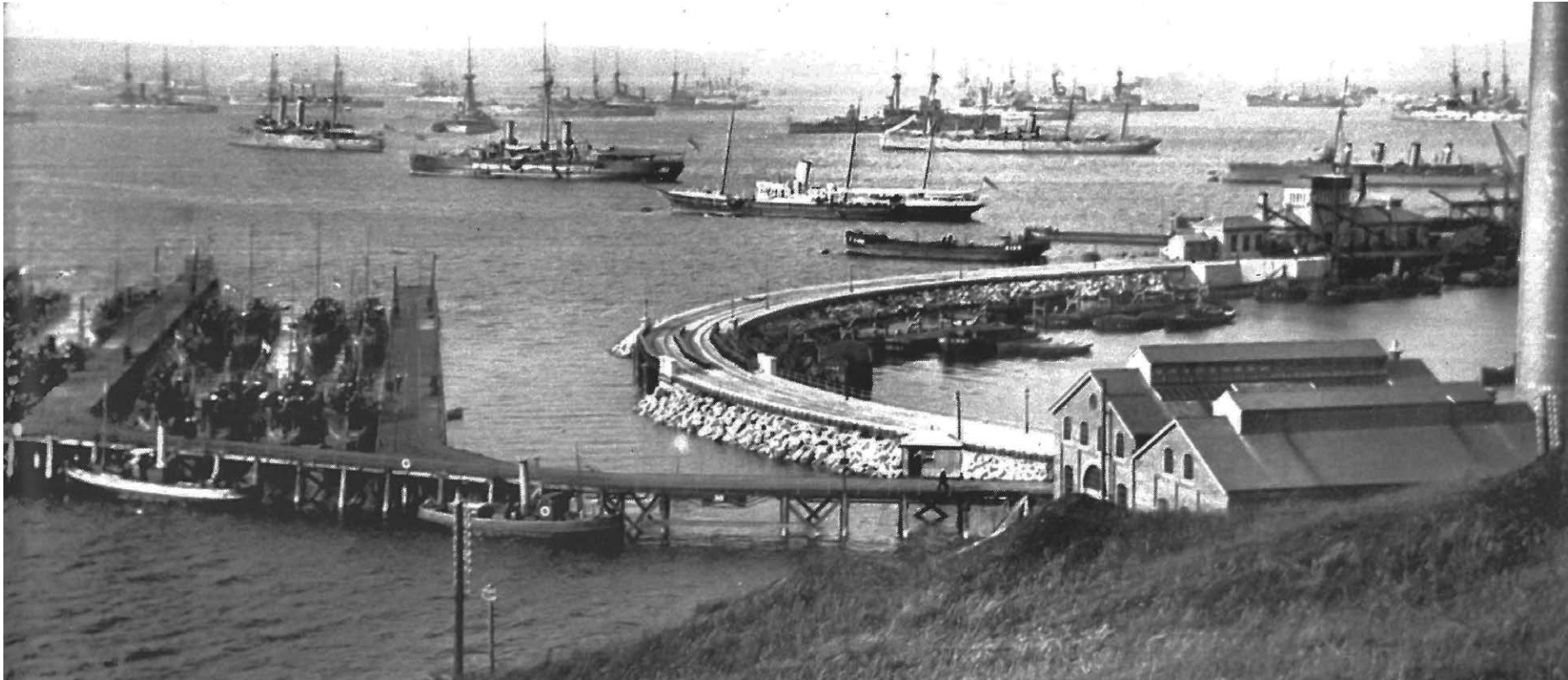
Fig. 36: Portland harbour Review of the fleet, 1912 torpedo boat pens (left) and electricity sub-station (right). Note transitional form of Royal navy ships with both masts and steam funnels. (Morris)
