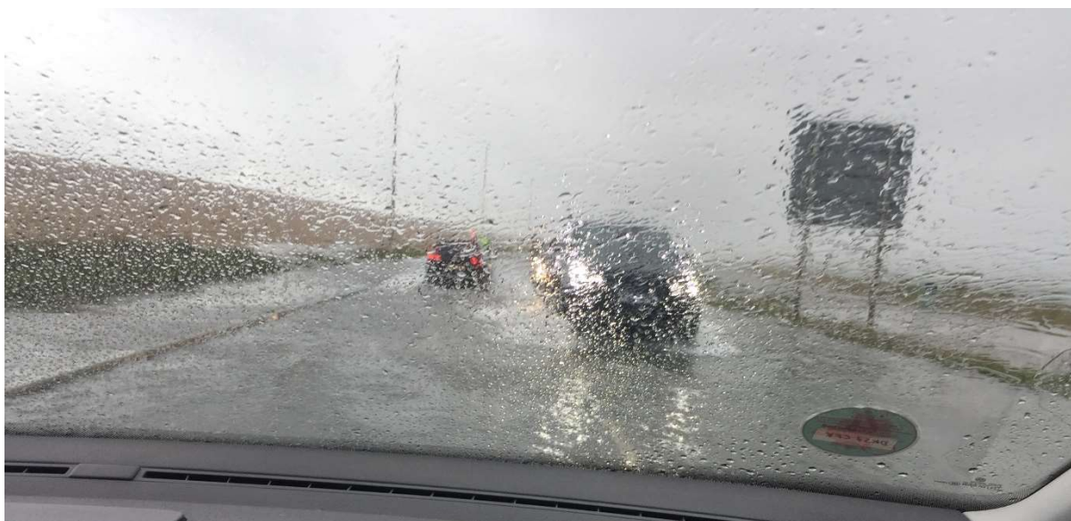
Fig 6: A354 completely inundated 2 nd Nov 2023 Island cut off for hours. photo SPWI
