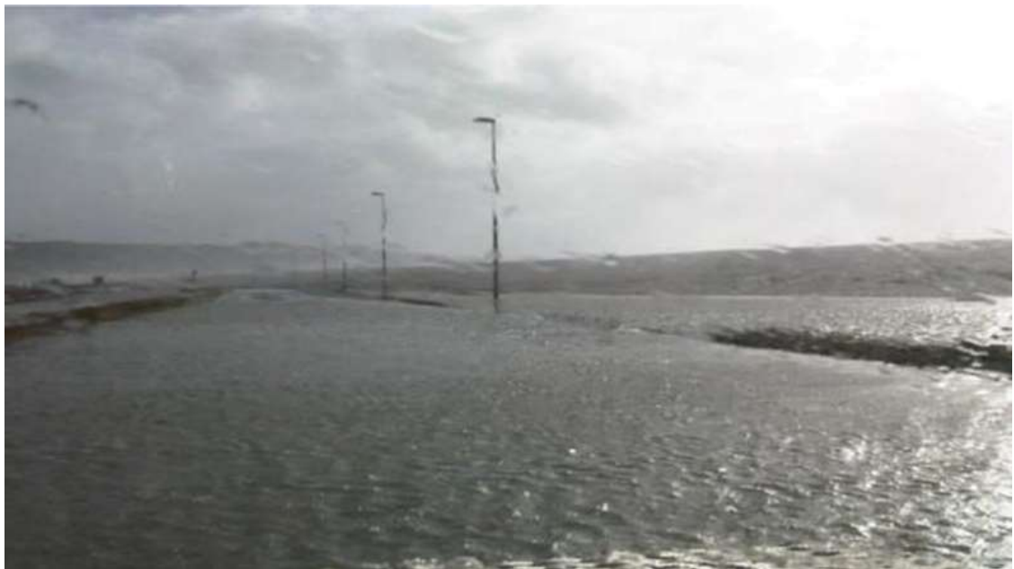
Fig 5: A354 completely inundated 5 th Feb 2014 Island cut off for hours. photo Grant Armfield C.Eng
