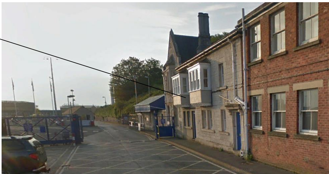
Figure 28. 1, Castletown, the only building in Castletown constructed of Portland Stone, an integral part of the Victorian operation of the harbour and port, listed grade II
