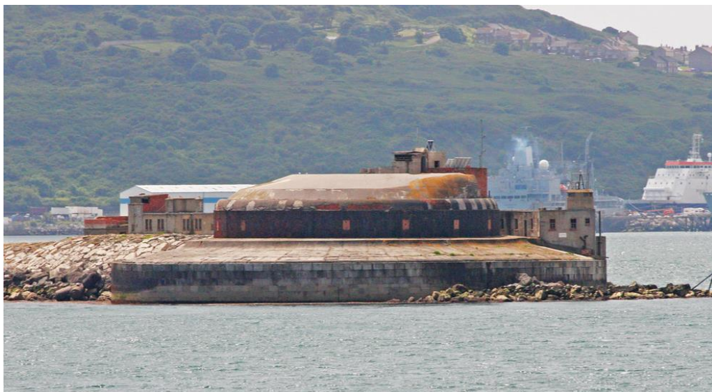
Figure 13. The outer breakwater seaward fort with the site of the proposed ERF in the background
