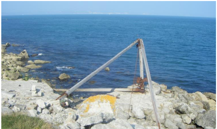
Figure 4. Durdle Pier with the C19/early C20 crane used for stone then for lowering fishing boats into the sea, the crane was lost in the 2014 storms © www.portlandhistory.co.uk
