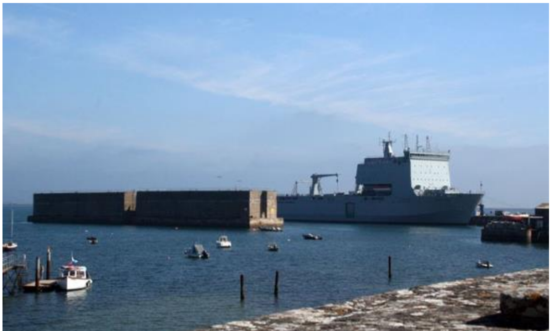
Figure 19. The grade I listed caissons viewed from the west
