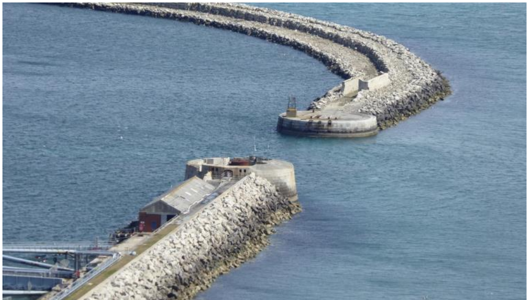
Figure 12. The fortified seaward end of the inner breakwater in the foreground. Outer breakwater extending in the background
