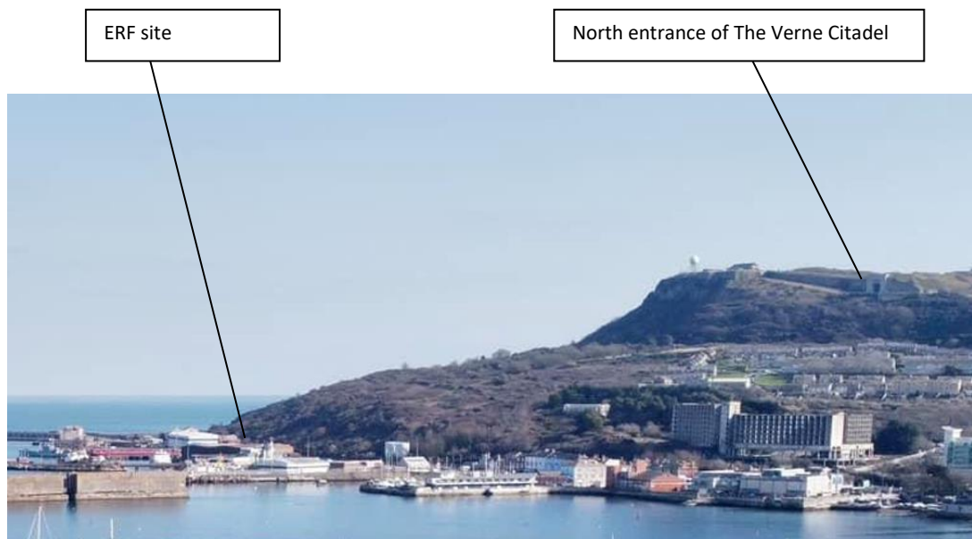
Figure 37. The huge northern gateway of The Verne that will have its apparent scale reduced further to the presence of the massive ERF in the harbour below; the harbour which the citadel was developed to defend
