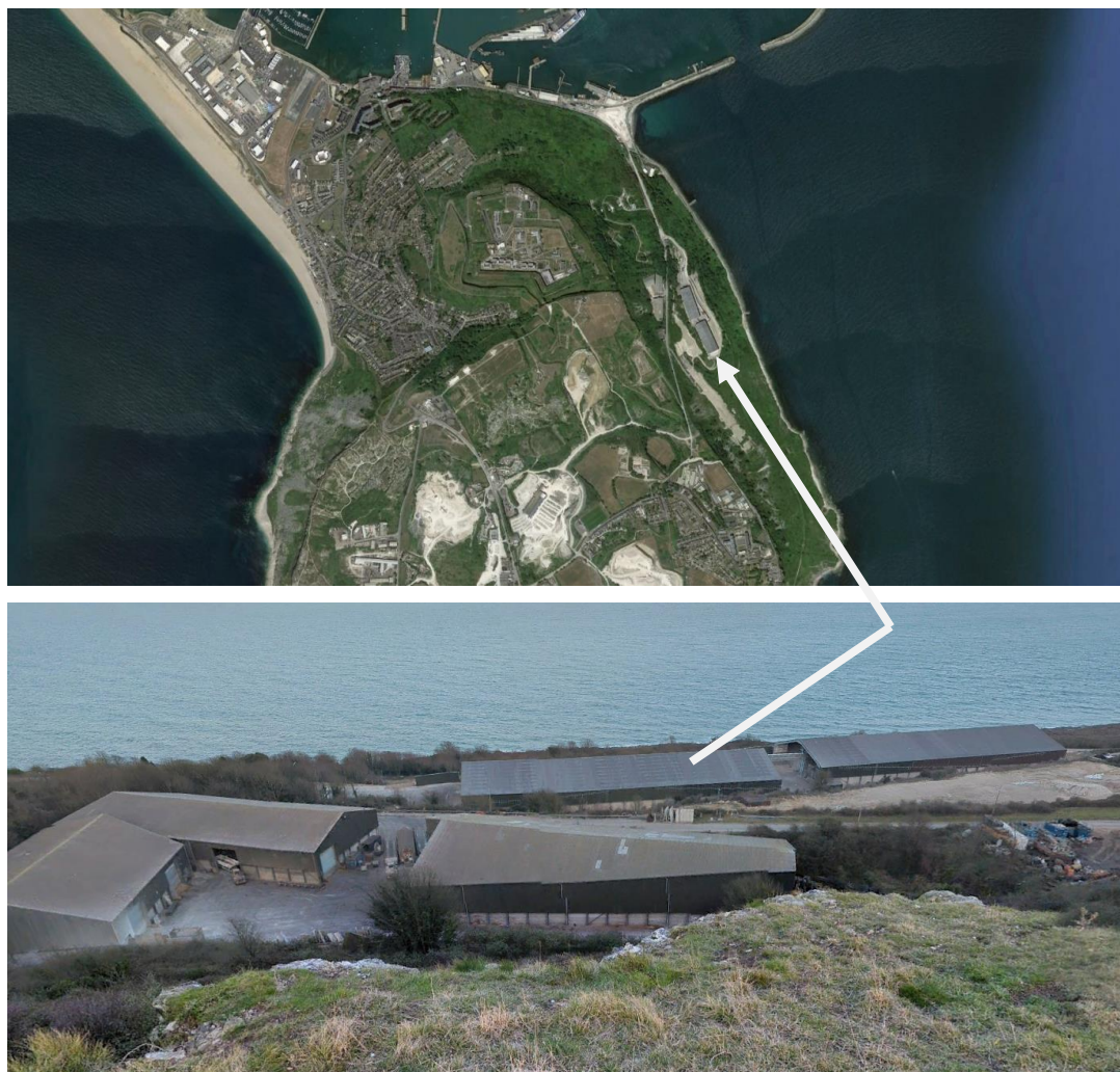
Figure 40. The well conserved east coast of Portland where the historic stone export piers are located. Top – aerial photographs showing the east coast © Google Earth. Bottom – the low, but large, portal frame building that are the on development along the east coast
