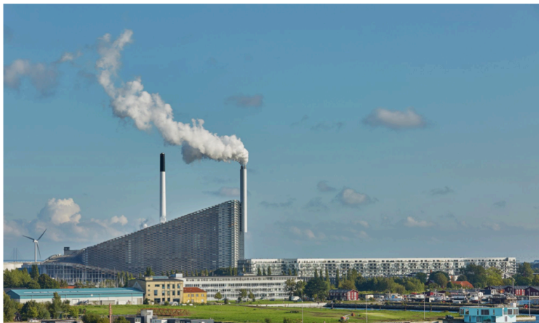
A waste-to-energy power plant operates in Copenhagen, one of many in Denmark | Image via iStock
