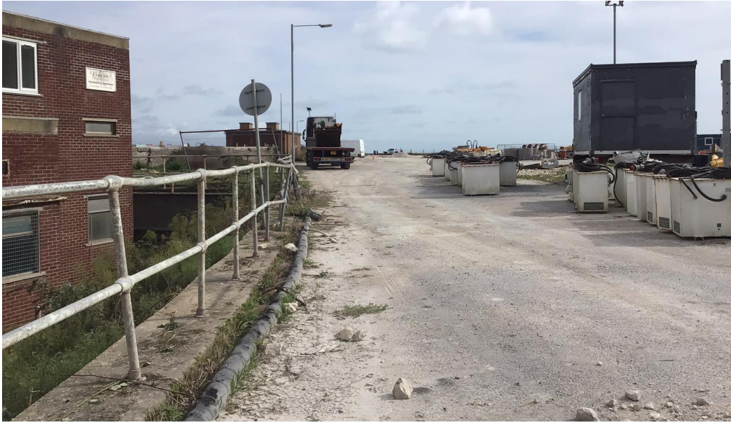
View from the Dockyard Offices towards the Inner Breakwater
