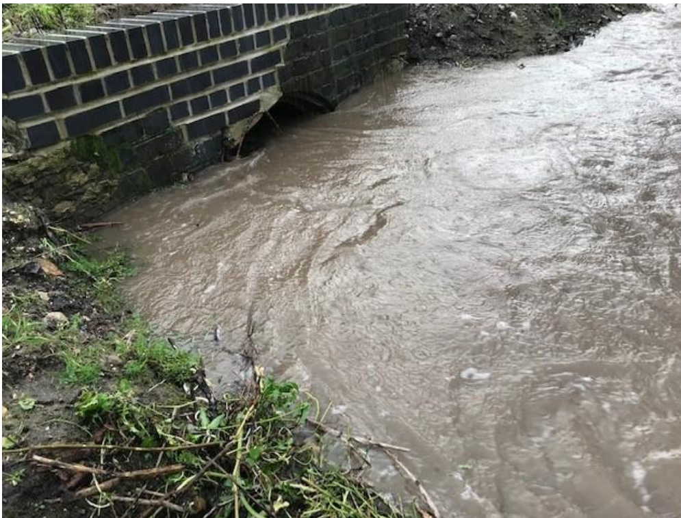
Culvert under railway embankment, Malthouse Meadows
