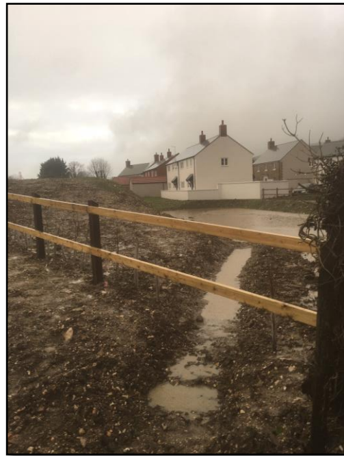
Photo 3 - Cut through at Malthouse Meadows
