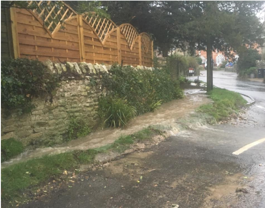
Elevated western channel, looking north-east towards front Street
